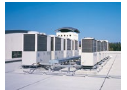
Outdoor units of multi-air-conditioning systems for buildings
