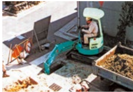
The Vi015 excavator
