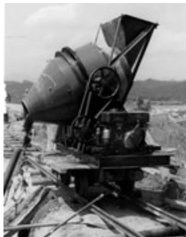
A yokosui engine used to power concrete mixers
