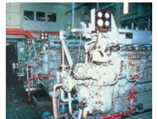
Cogeneration system at the Showa Station in Antarctica
