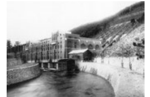
The Uji power plant of Ujigawa Denki (completed in 1913)
