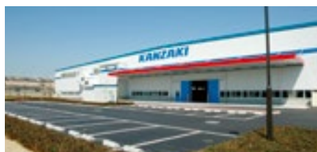
The head office's new plant at Kanzaki Kogyukoki (2004)
