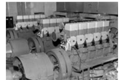
Large engine-generators supplied to the Cosmic Ray Observatory of Tokyo University on Mt. Norikura
