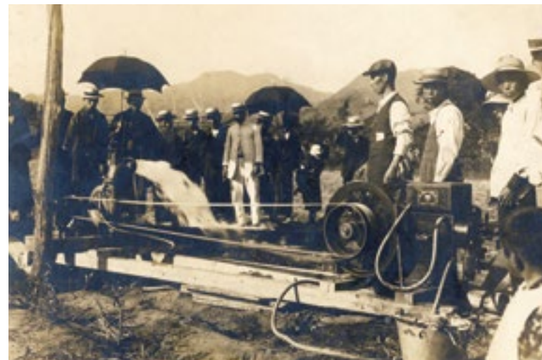
Water pump powered by a Yanmar oil engine (Sasayama, Hyogo Prefecture, 1925)
