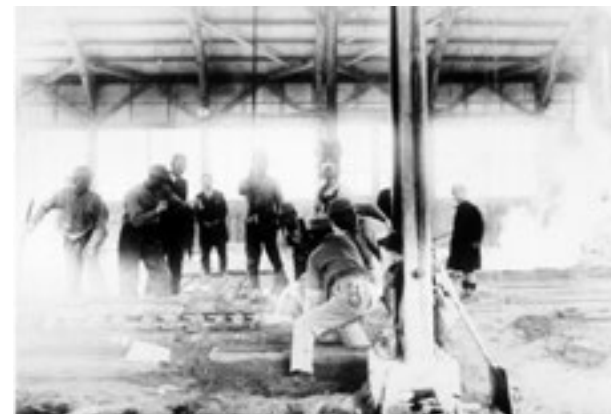
Start of operations at the die-cast plant
