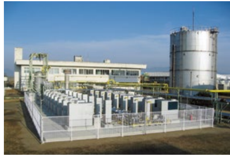
Saga Sewage Treatment Center (2011)
