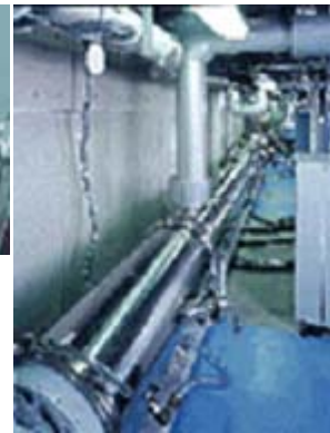
Diesel engine exh. gas measuring equipment (dilution tunnel)
