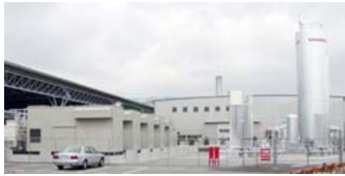
Overall view of gas cogeneration facility
