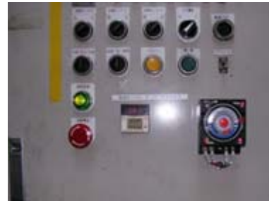
Power control panel with weekly timer
