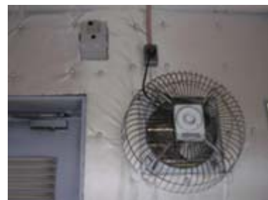
Ventilation fan with thermostat
