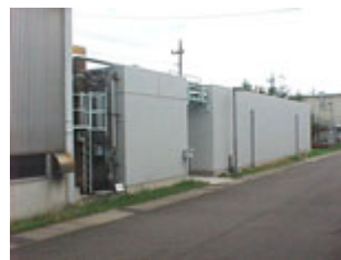
Waste treatment facility of Biwa Plant, (new Nitrogen Removal Equipment, right)
