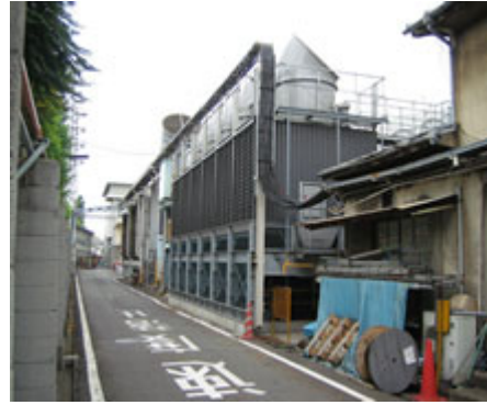
CW Pit & Cooling Tower of Amagasaki Plant In order to maintain the temperature of the CW pit below 30°C, industrial water was fed into the pit in the past. This feeding of industrial water was much reduced by cooling in the cooling tower.
