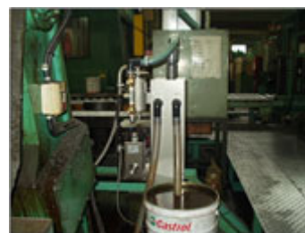
Floating oil/water separator added.
