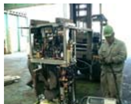
Recovery of coolant (unit turned for easy recovery)
