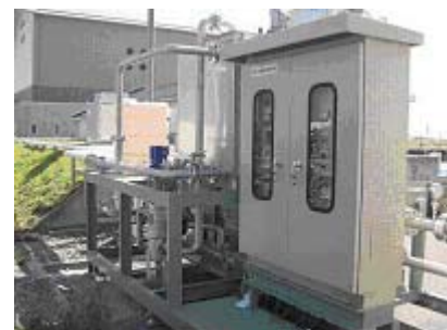
Sludge Reduction System
