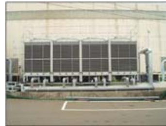
Change of cooling tower to supply CW water for use with test operation
