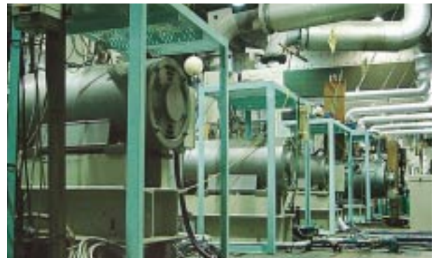
Power generation section
