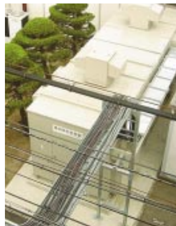
Power regenerator of the Nagahama Site
