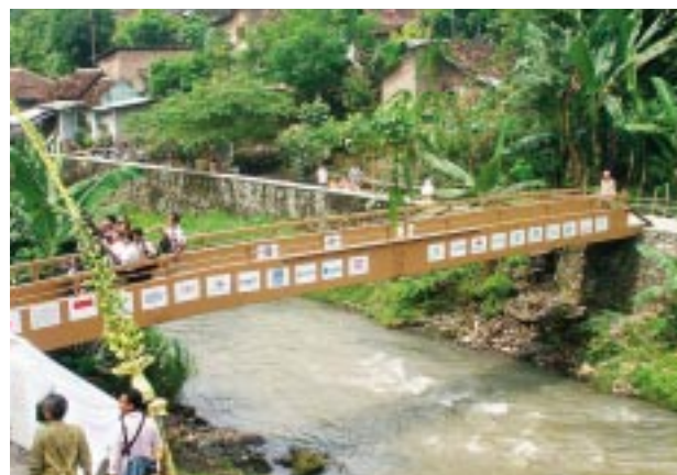
Relocated pedestrian bridge
