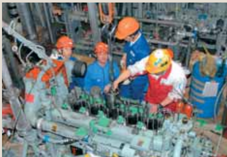
Overhauling a generator
