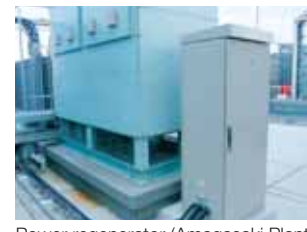
Power regenerator (Amagasaki Plant)
