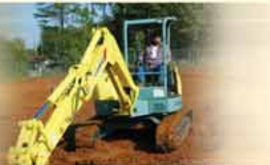
A mini-excavator, frequently used for infrastructure development in urban areas
