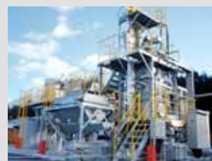
300 kW biomass gasification cogeneration system
