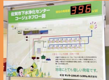
Display of power generation
