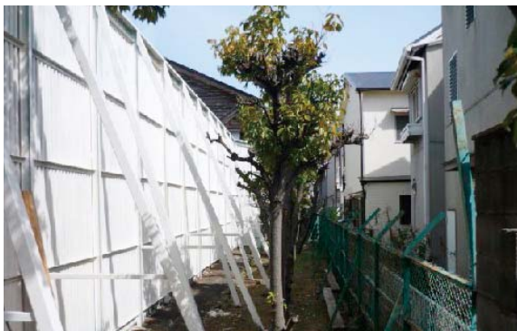
A sound barrier (painted in consideration of local scenery)
