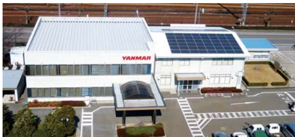
The solar panel installed on the roof of the annex of the Amagasaki Plant.
