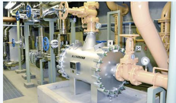
A sludge heat exchanger that exchanges the heat of warm water from the cogeneration system
