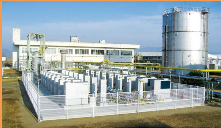
16 Biogas Micro Cogeneration System units
