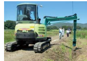
Contaminated soil that has built up in cultivation ditches is removed using a small backhoe.
