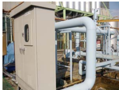
Cooling water pump motor (Tsukaguchi Plant)
