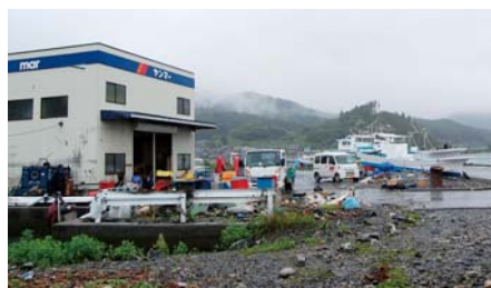
Temporary repairs at a plant
